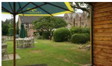
District heat main was laid across the hotel garden,
