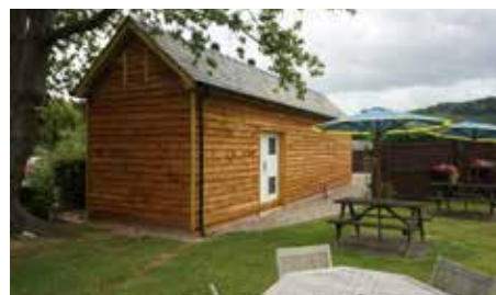
The plant room was finished with wood cladding with a reclaimed Welsh slate roof.
